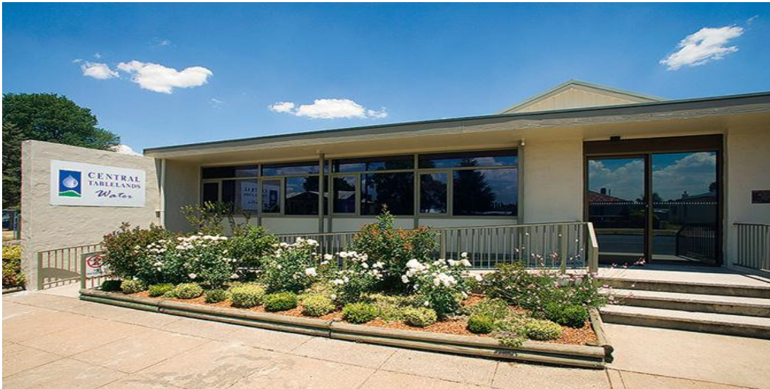
Central Tablelands Water – Administration Office - Blayney
