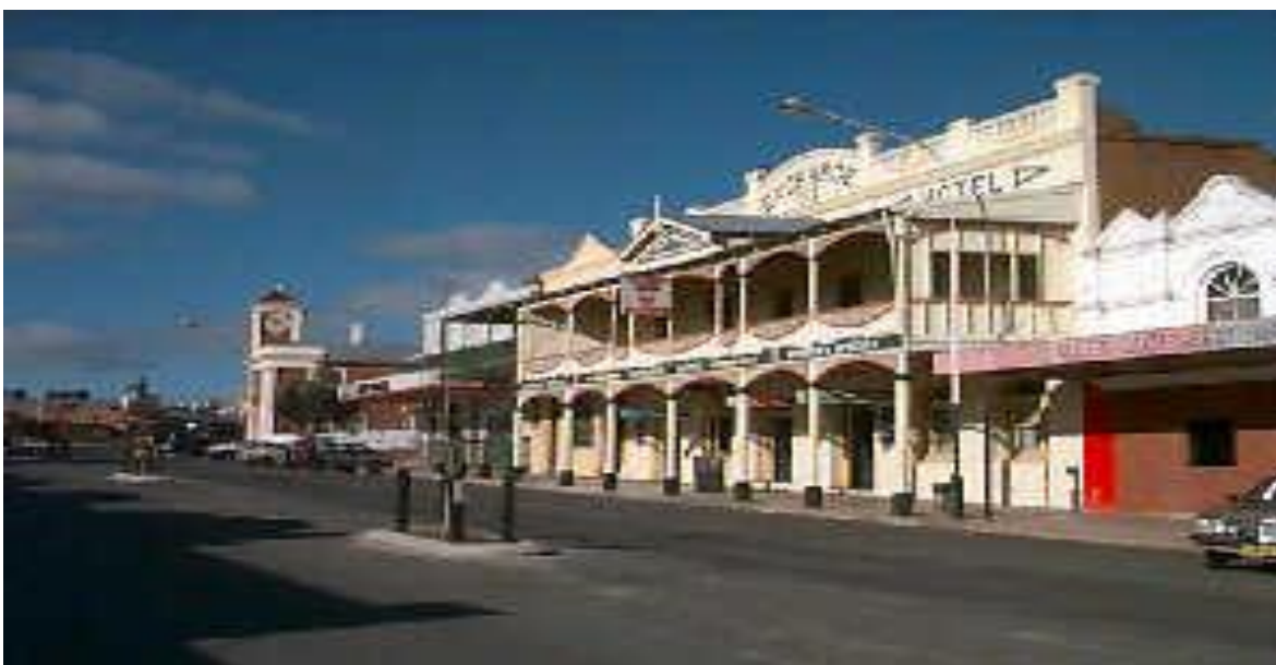
Town of Grenfell
