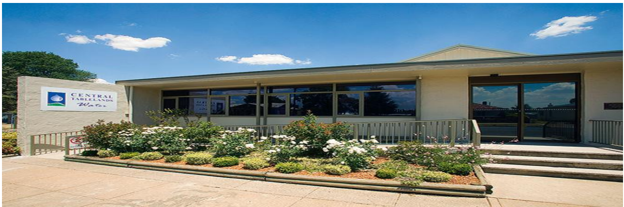
Central Tablelands Water – Administration Office - Blayney
