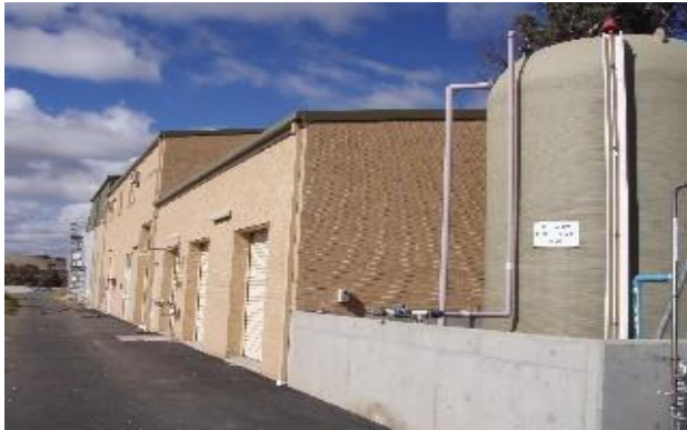
Carcoar Water Filtration Plant
