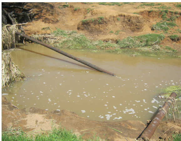
DAMAGE TO CTW TRUNK MAINS MARCH 2012
